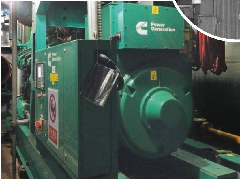
Cummins lean-burn generator sets were used, using natural gas to generate electricity and at the same time recover the waste heat to satisfy the demands of central airconditioning and heating in the airport.
