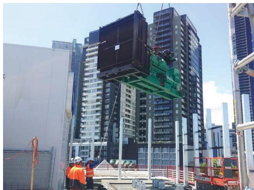
Two special challenges on the project were vibration and noise. The generator set was to be mounted at roof level, actually spanning the refurbished original building and the new building constructed at the rear of it.
